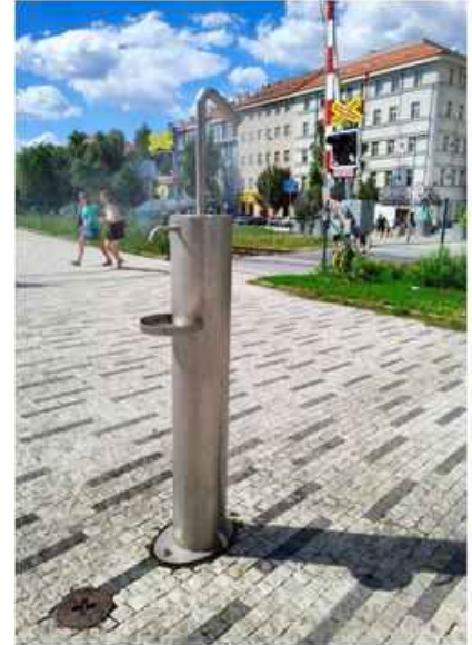
Photo 2. Prague waterworks and sewerage
